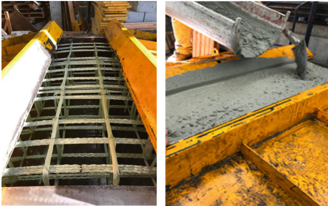
Fig. 1. GFRP reinforcement detail and concrete cast
