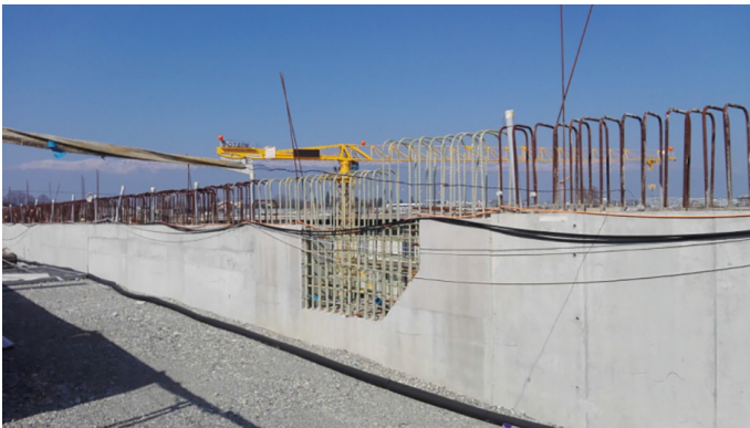
Fig. 15. GFRP reinforcements in a portion of a concrete wall
