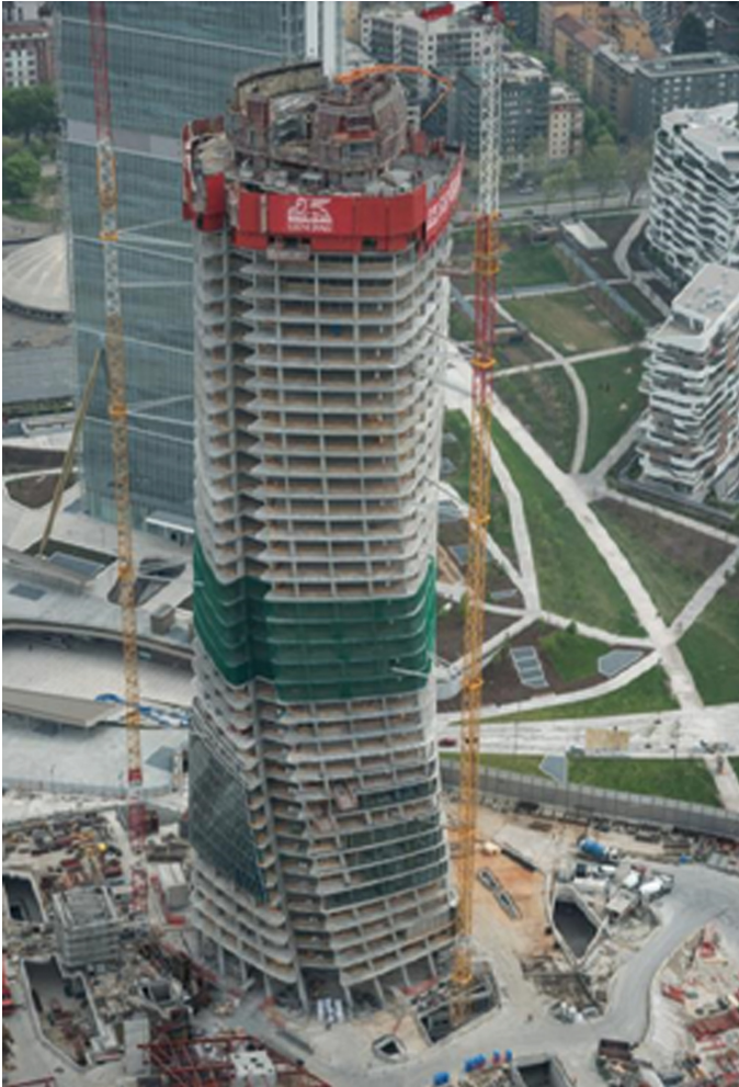
Fig. 2. The concrete structure rising
