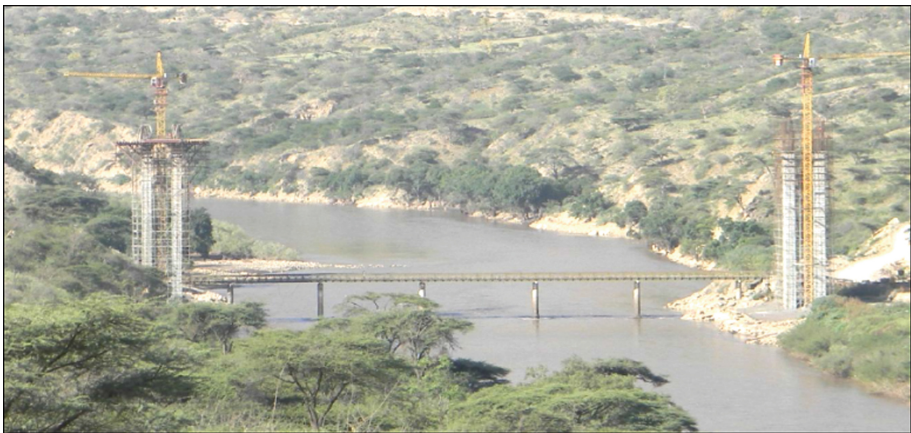
Fig. 8. View of the bridge under construction
