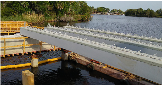
Fig. 9. HCB during installation.
