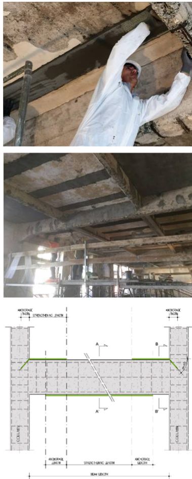
Fig. 9. Flexural strengthening of beams and slabs.
