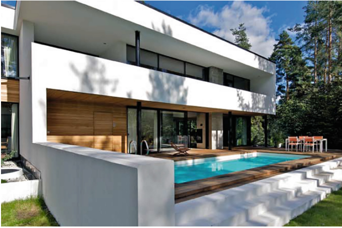
Fig. 5. Swimming pool realized with non-metallic reinforcement
