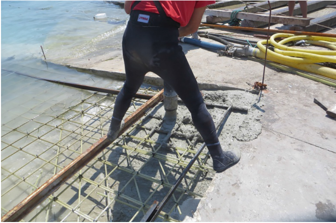
Fig. 13. Casting of the slab
