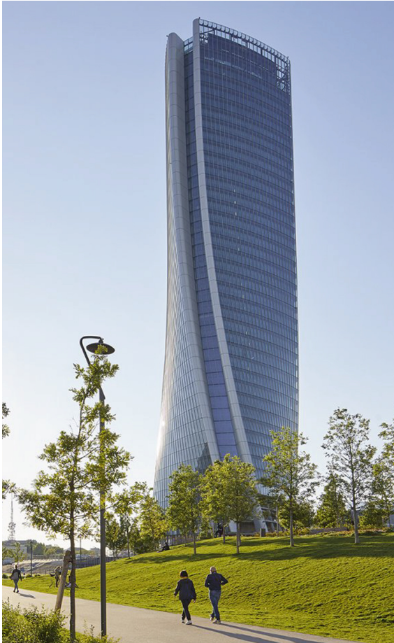
Fig. 1. The tower completed
