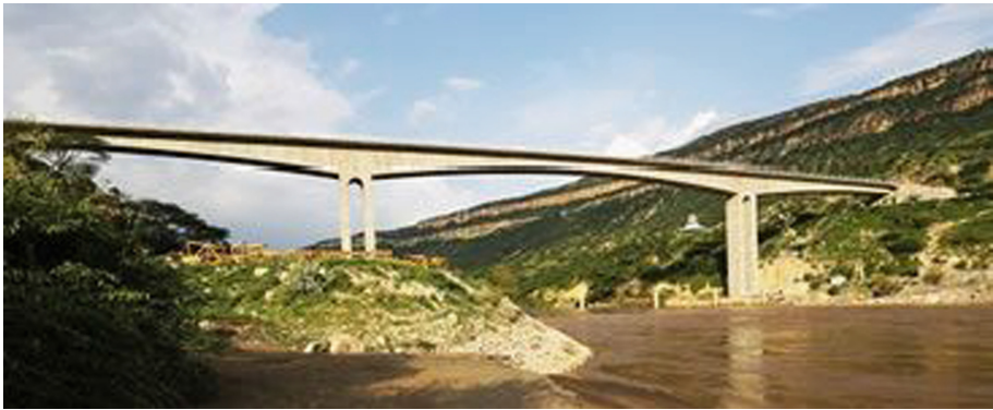
Fig. 7. General view of the bridge
