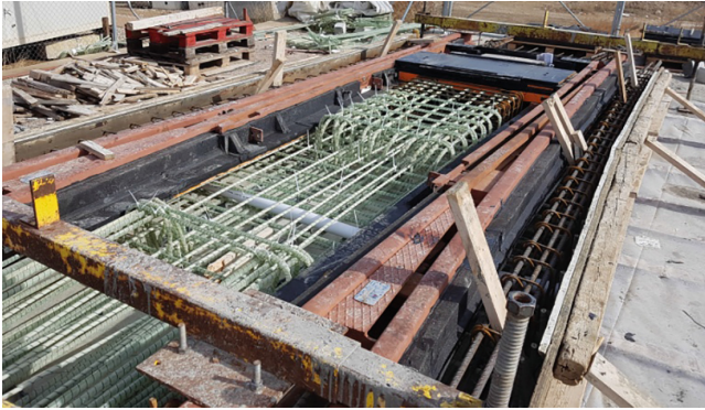
Fig. 3. GFRP reinforcing cage assembled on the track beds
