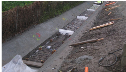
Fig. 3. Installation of the reinforcement meshes
