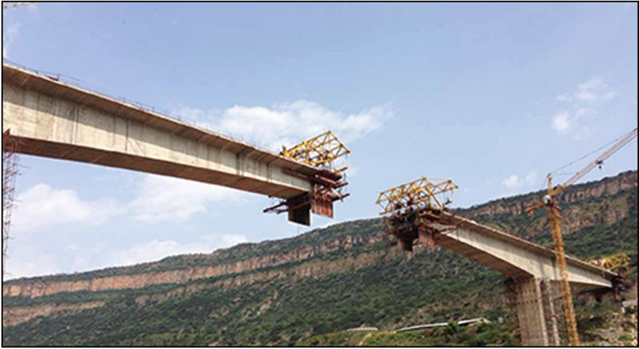
Fig. 9. View of the bridge under construction
