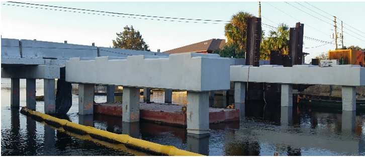
Fig. 7. Pile bent cap after demolding.
